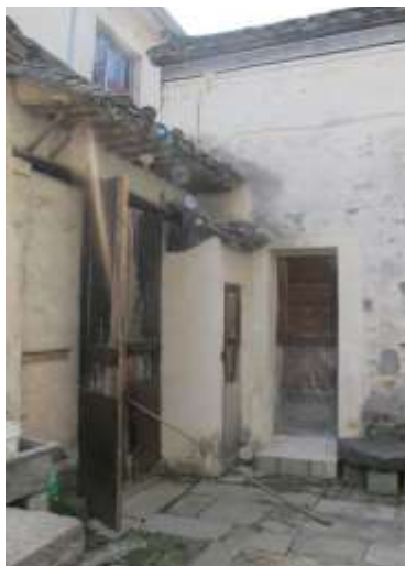
Figure 2-6 Toilet added to Chunhui Hall in Shangshuizhen
