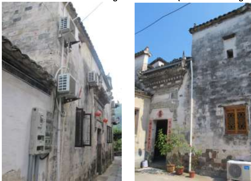
Figure 2-15 Added window and changed external wall (Left is W7 and right is W3)
