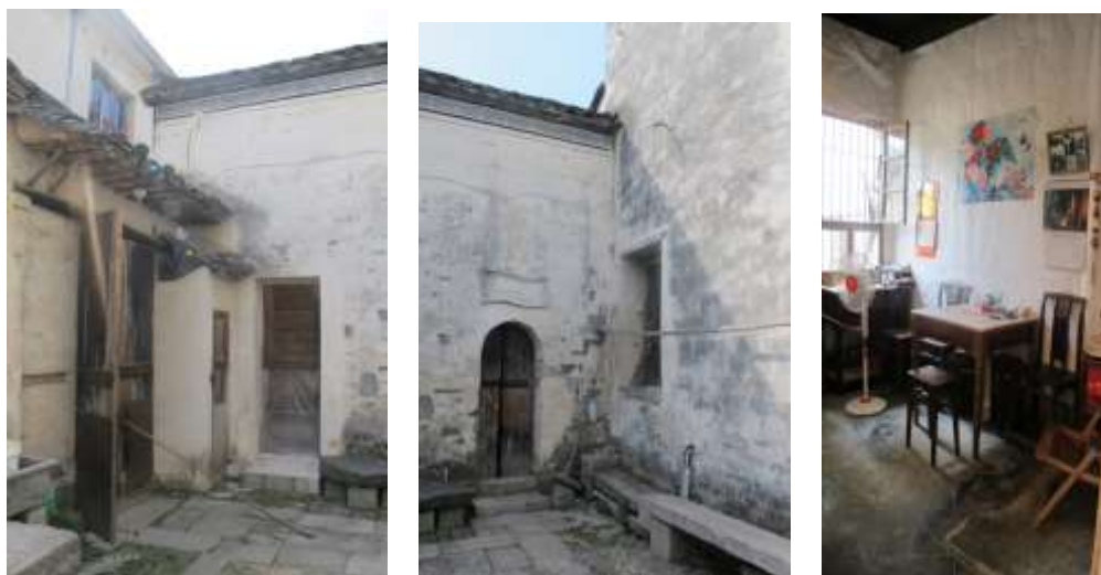
Figure 2-14 Toilet and bathroom (left and middle) in the annex and lounge changed from a silkworm shed (right)
